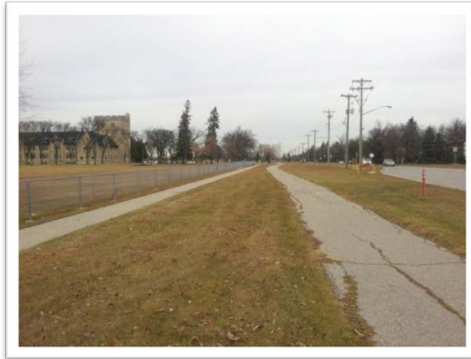
Existing pedestrian and cycling facilities on Shaftesbury south of Grant
