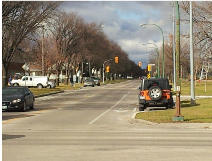
Harrow bicycle lanes with parking bays
