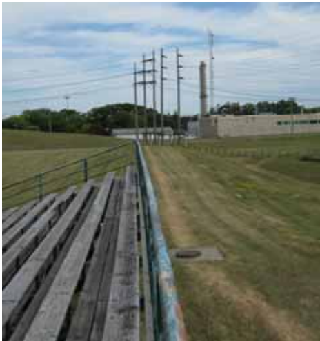
Looking east towards the McPhillips Pumping Station from the grandstand on McPhillips Athletics Grounds
